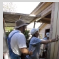
Matt Sailors (l.) and Tracy Byerly replace outside panels.
