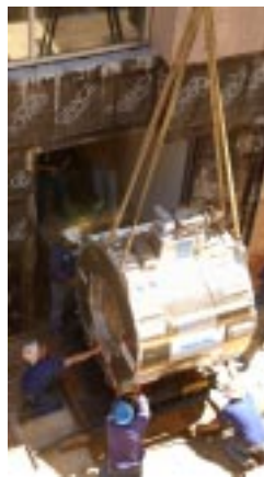
Workmen guide the Tesla installation.
