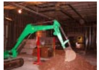
Track excavator at work underneath terrazzo floor in basement.
