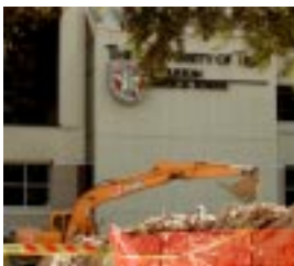
Front end loader at work on the Fannin side berm project.
