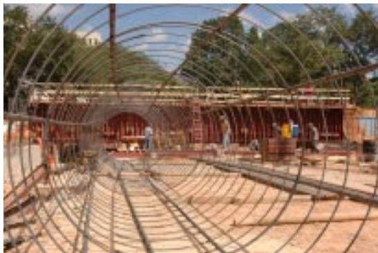
Structural work commences on the RRF in this June 8 photo.
