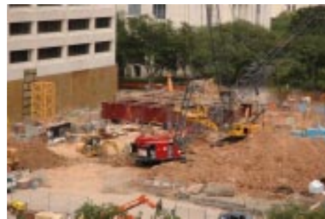
Heavy machinery gets RRF construction moving June 15.
